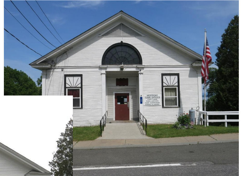
Façade before restoration
